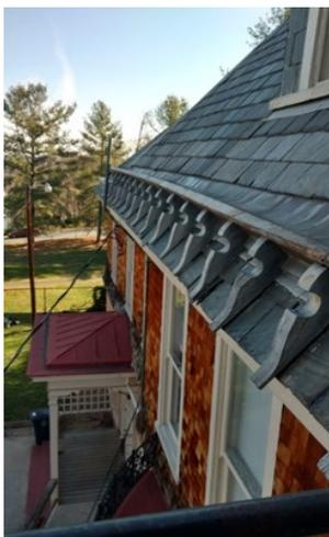
further examination, wooden structural members under the hidden gutters and supporting dormers were also deteriorated. Recently, active water intrusion began in the ceiling of the hall and office space on the second floor. This is ongoing and causing additional damage to structural wood members in
